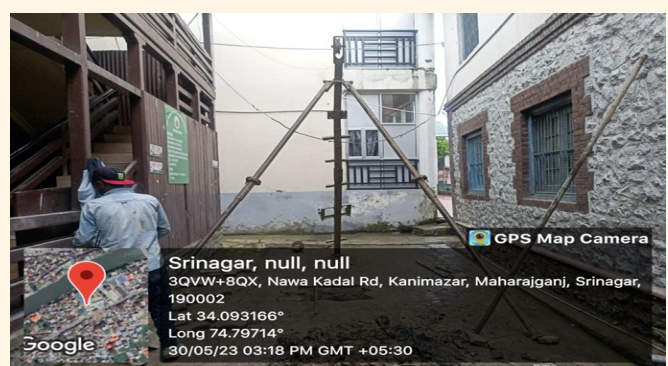
Soil Testing in Progress in connection with the construction of academic cum establishment Block.
