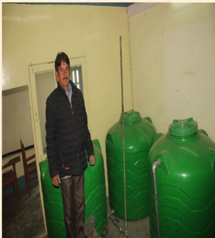
Replacement of old iron water tanks by plastic tanks in the old academic block
